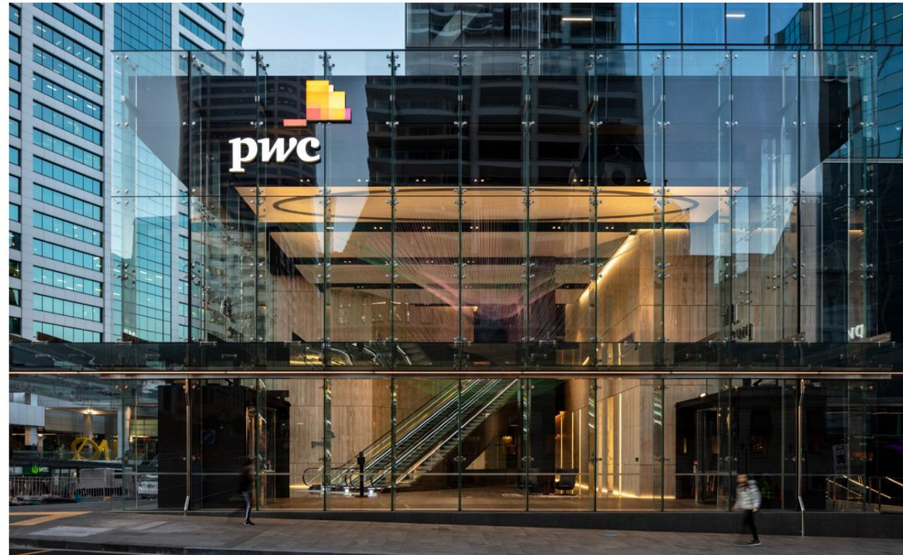
**TOTALVISION IS A HIGHLY ENGINEERED FRAMELESS GLASS FACADE. THIS TOTAL VISION SYSTEM UTILISES STRUCTURAL GLASS FINS AND FITTINGS LIKE STAINLESS STEEL SPIDER FITTINGS IN ORDER TO OFFER UNENCUMBERED VIEWS AND A STUNNING AESTHETIC.**
