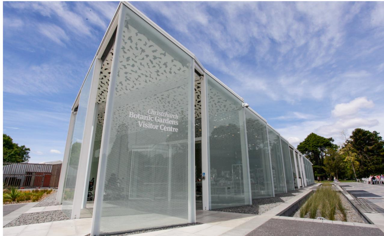
**KERAMO IS GLASS THAT UTILISES A CERAMIC FRIT PATTERN. IT IS OFTEN KNOWN AS “FRITTED” GLASS AS IT USES CERAMIC GLASS FRIT MIXED WITH SPECIAL ENAMEL PAINT AND COLOUR OXIDES.**
